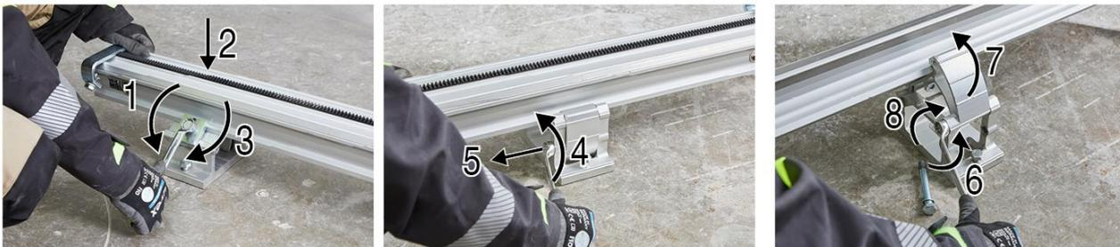
4. Fit the track onto the track supports.
