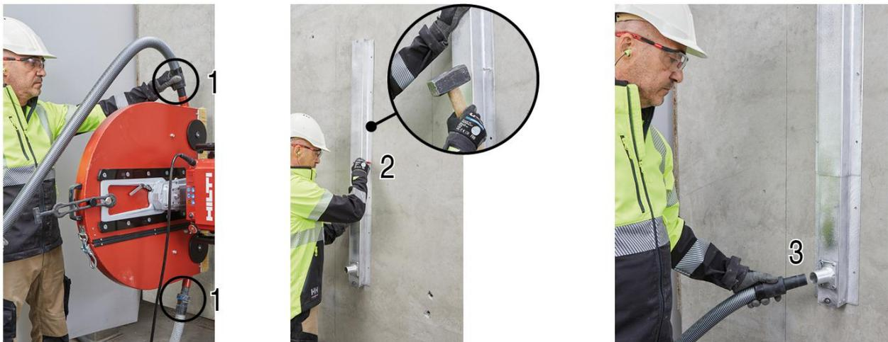
1. Install the BG 65 blade guard (dry cutting).
